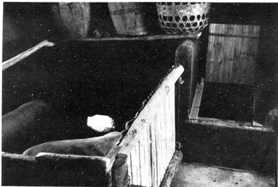
Plate 18. Inside a pigsty at Liang Chu People's Commune (Zhejiang Province) showing the household latrine situated in the same building. The latrine and pig pen connect directly to a biogas unit beneath the floor.
