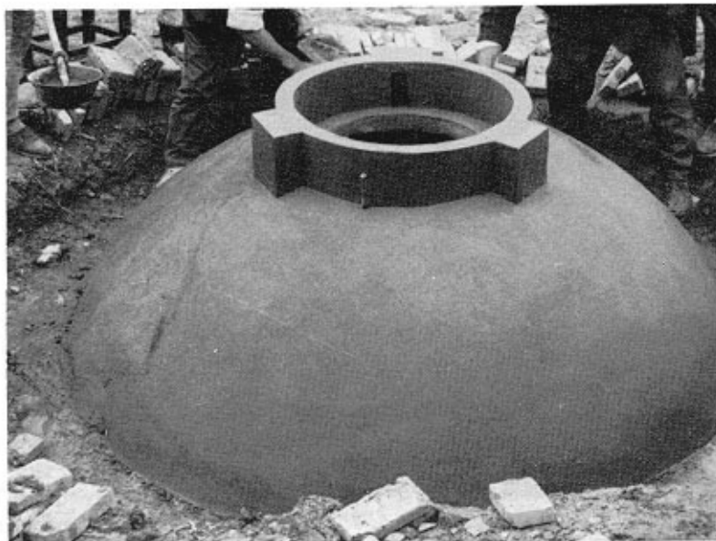
Plate 24. The dome of the biogas unit shown in Plate 23 when completely finished and awaiting the manhole cover. Note the strengthening collar on the top, fitted with slots for bricks to hold the cover in place. The gas outlet tube can be seen just in front of the collar.
